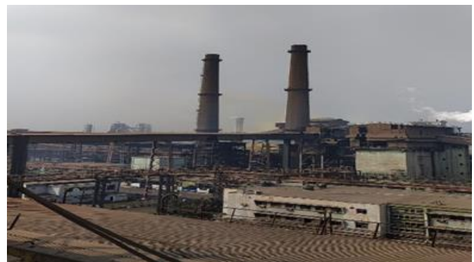
Fig. 1 BHILAI STEEL PLANT (RCC Chimney)
